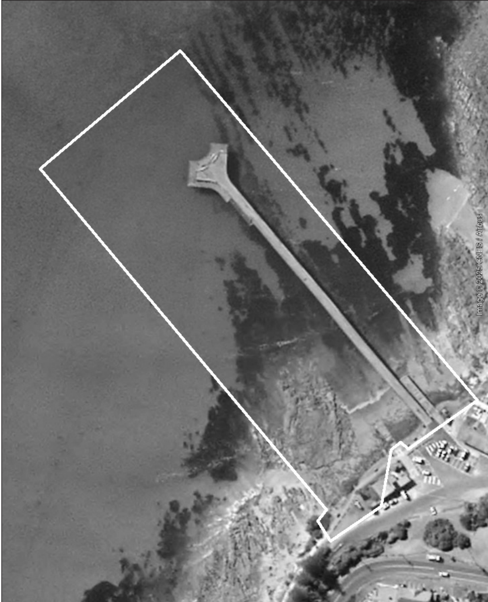
Attachment A – Lorne Pier – Access Prohibited
