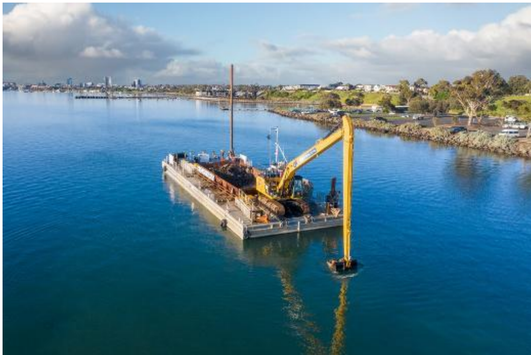
Figure 2. Basalt rocks being deposited to form 'Merv's Reef', St Helens, Geelong.
