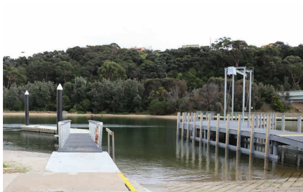
North Arm: The new-look facility includes a new concrete boat ramp and apron and a floating pontoon to the west of the ramp. A new fixed eastern jetty was installed which relocated the fishing gantry to the water's edge, making it easier to weigh in large fish.
