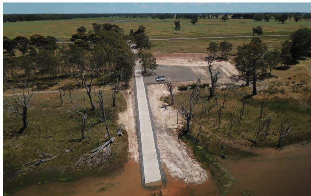
Toolondo: The boat ramp was replaced with a concrete surface and additional car parking was provided.
