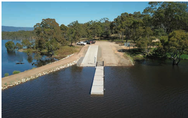
Lake Lonsdale: A new concrete ramp lane and rock beaching was installed at Lake Lonsdale to double capacity at the boat ramp.
