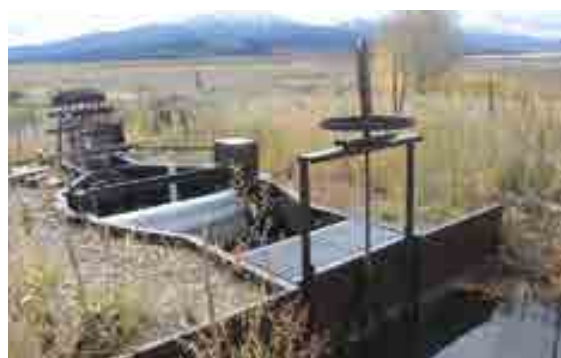
Example of a rotating drum irrigation diversion screen
